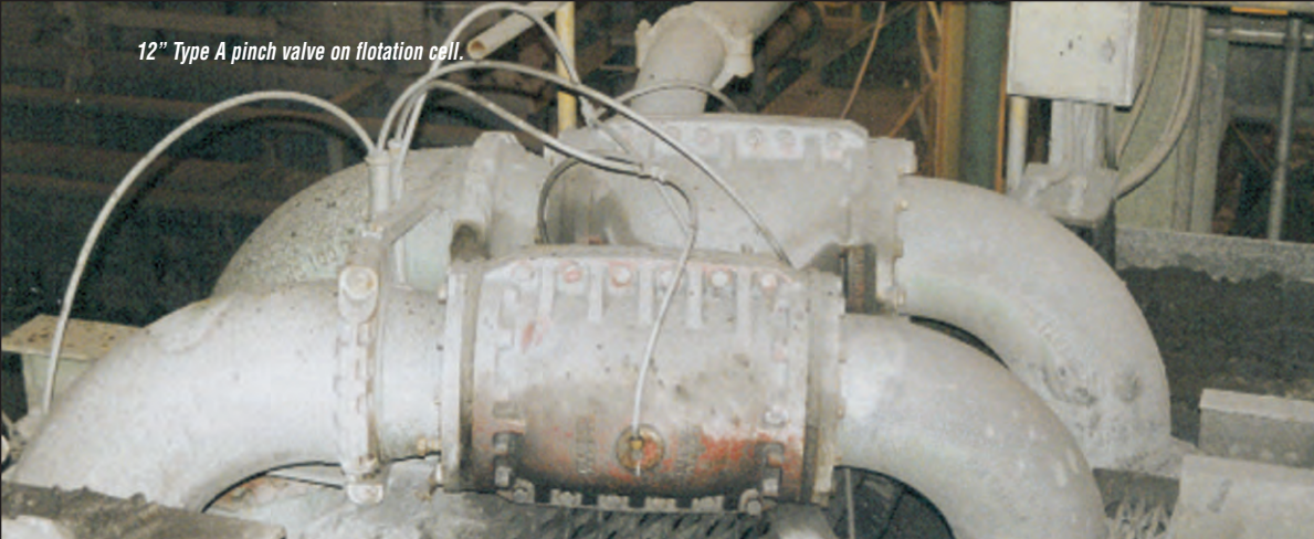
Control pinch valve maintains level on this thickener underflow system at the Escondida Mine in Chile.
